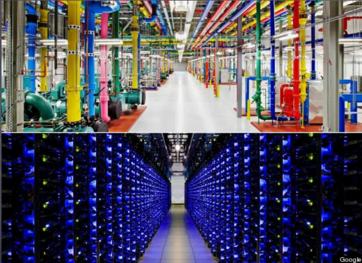
Google Data Center
